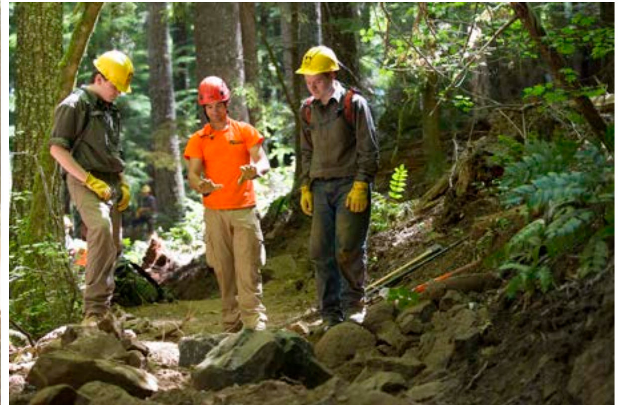
Whistle Punk construction specifications reflect the conceptual plan and design guidelines to produce the desired experiences. In this case, rock was imported and placed to provide more technical challenge than native materials could provide.
