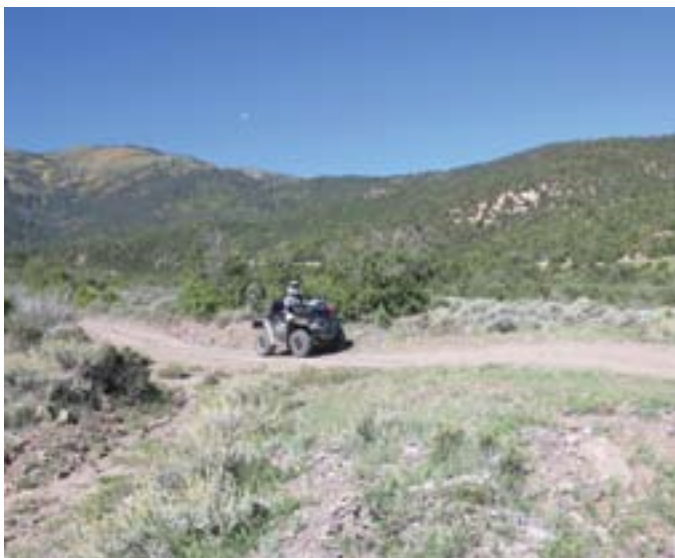
The flatter the trail grade, the more functional and durable the dip will be. This one is perfect: long, flowing, and deep.
