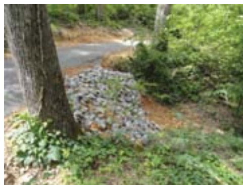
A blanket of cobble rock at the drain point of this trail protects the fillslope from scour and erosion. This protection is especially important where there is the potential for high volume and high velocity water flows.
