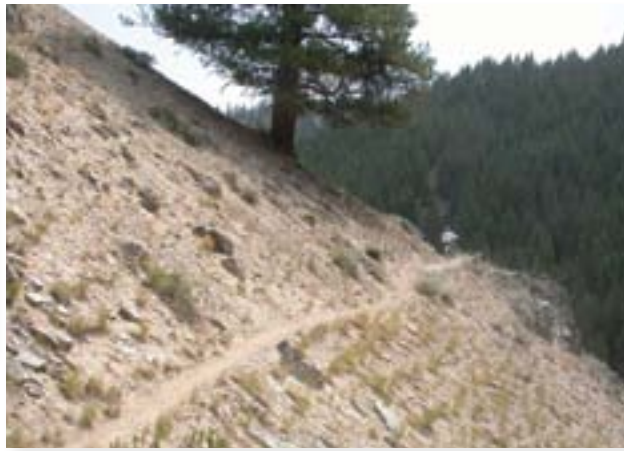
A narrow tread on an open slope like this reduces the margin for error, reduces the riders' perception of safety, and therefore increases the feeling of challenge.
