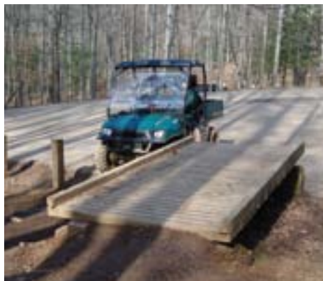
This is a nice ramp, but weather and tire action are eroding the approaches. They need to be hardened to keep it functional.
