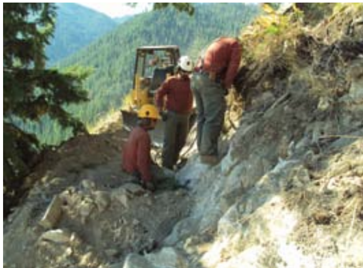
The deeper the cut, the higher the likelihood of encountering solid rock. Having air tool capabilities makes this less of an obstacle.
