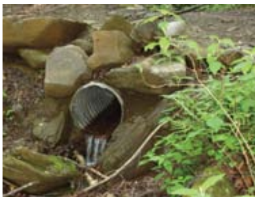
There are drawbacks, but culverts allow water to drain under the trail and keep the tread dry.
