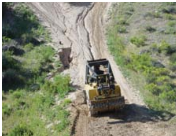
This trail is in obvious need of reconstruction. The tread watershed is too big and too much water is draining at this point.
