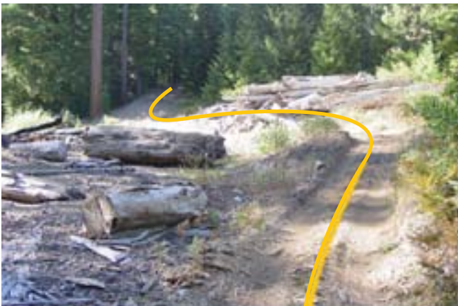
The designer took advantage of this old landing to leave the road corridor to provide sinuosity and drainage.
