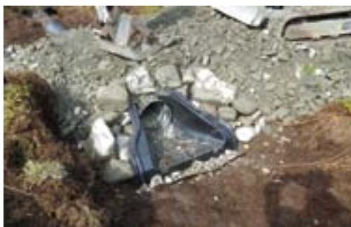
A flared inlet and headwall are being added to this culvert to help funnel the water into the inlet. Though a small diameter culvert like this may be adequate to handle the flow of water, it is very hard to keep cleaned out.
