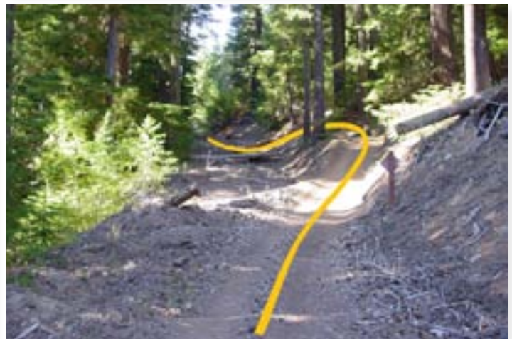
Here the trail pitches up to the top of the cut bank, around some trees, and then back down again. Though short, it provides diversity for the rider, sinuosity, and drainage.
