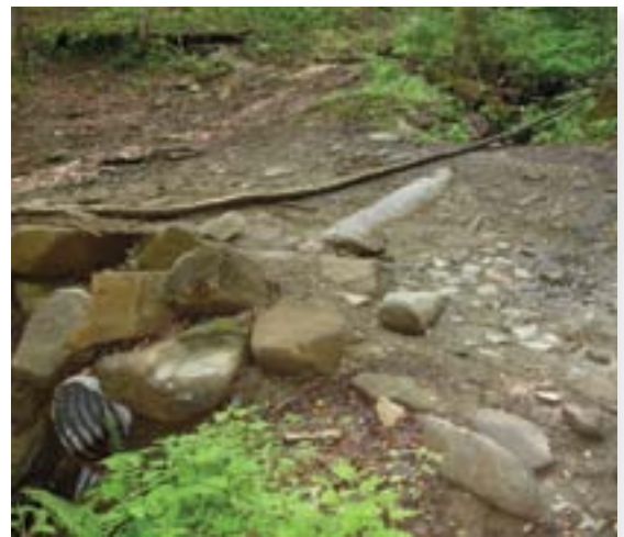
The top of this culvert has been damaged and will eventually break which compromises the integrity of the structure and increases agency risk.
