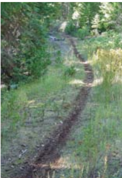
The designer took advantage of this old landing to leave the road corridor to provide sinuosity and drainage.
