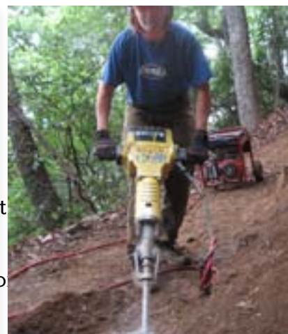
Pneumatic rock splitters clear away stubborn rocks in the tread.
