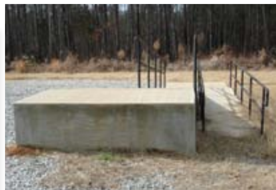
With the concrete and the railing, this ramp was expensive to construct. It is accessible, but the approaches in the gravel probably aren't. If the concrete truck is going to be there, why not pour a concrete parking pad and approach to the ramp?
