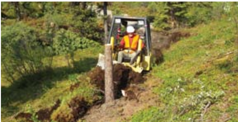
The dozer is removing the organic layer of vegetation and grubbing stumps. Note the high-cut stump for increased visibility and leverage.
