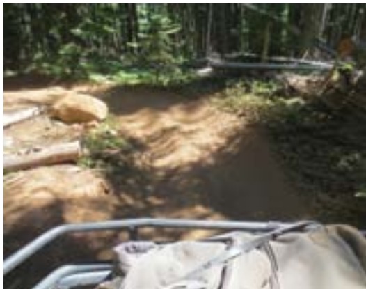
This is a new trail that was ridden in. The lack of a constructed tread has resulted in deep ruts created by compaction and displacement.
