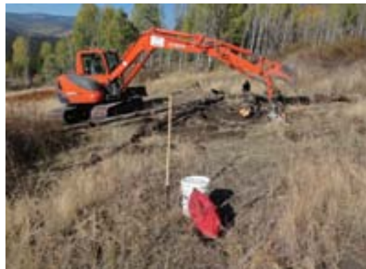
An excavator places debris and installs logs in a herringbone pattern to close off hillclimbs on a sensitive grassland. Note the hand-seeder and bucket of seed ready for immediate application.
