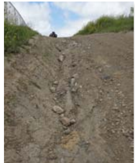
Due to a lack of training or awareness, maintenance personnel have bladed out the rolling dip at the top of this steep hill allowing water to run down and erode the slope.
