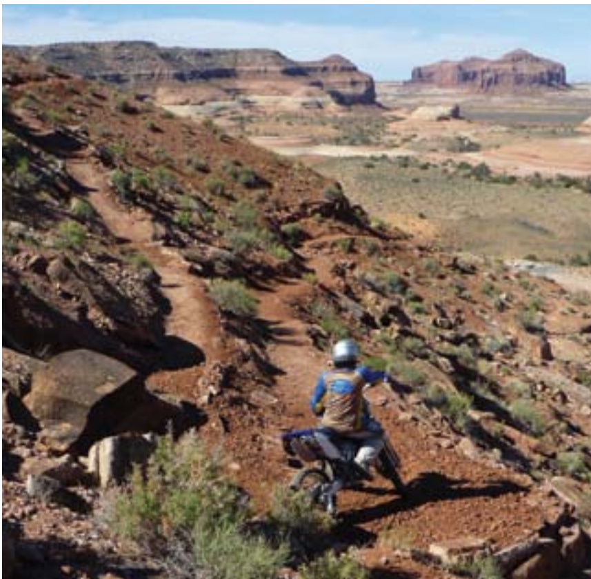
A nicely-designed switchback. Notice how the grade of the upper approach flattens off before the landing. This adds significantly to the rideability of the structure. The landing is long and wide to allow room for a smooth turn on a circular curve.
