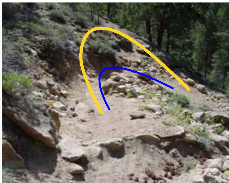
This structure has a nice circular curve, but no flattened approaches. Note the drain above and there's one below also which is good. It may have been better for drainage and rideability to use the top of the exposed rock as a flat area for the lower approach and part of the landing.
