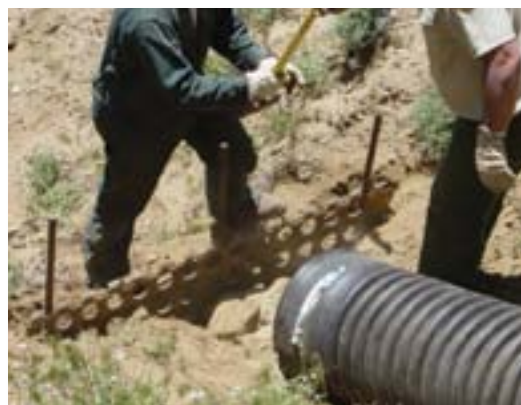
Installing an energy dissipater at a culvert outlet
