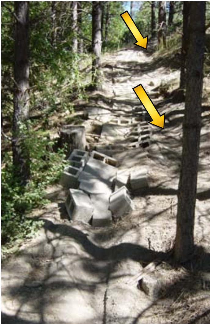
Poor bedding + no containment + movement = failure. You can see (arrows) where riders are going up the right side to avoid this installation.
