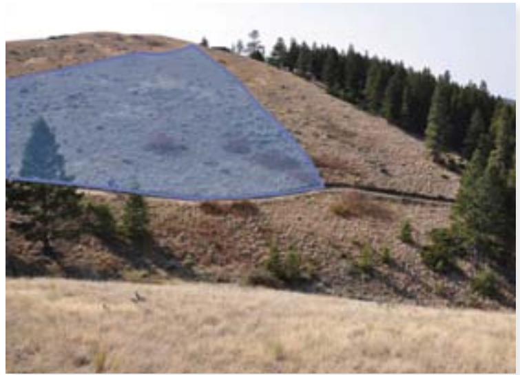
The height of the watershed above this trail is relatively low, but the topography is steep with low vegetative cover and exposed soils. The runoff potential here is high.
