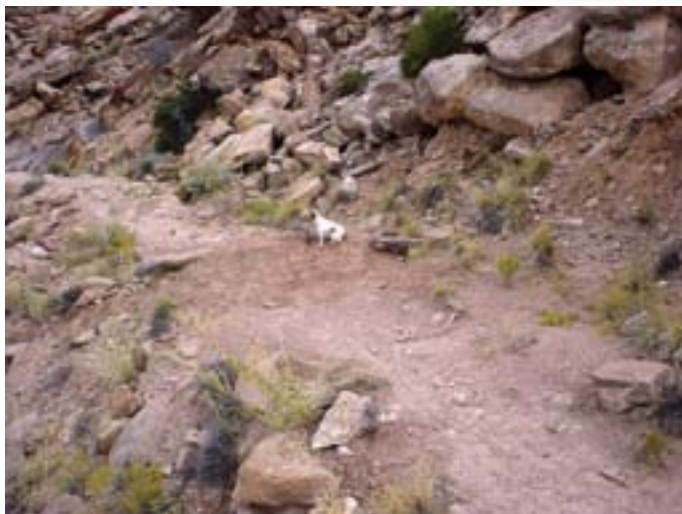
A newly constructed rock waterbar with a smooth approach. (Note: these will work if the rocks are large and well-embedded to resist the tire impact forces.)
