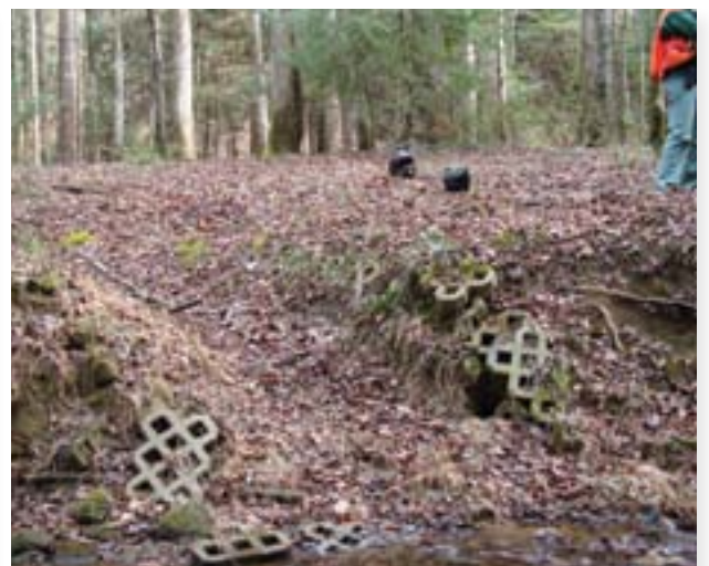
Poor paver installation in this stream crossing resulted in resource impacts. Cobble stone would have been a better choice.
