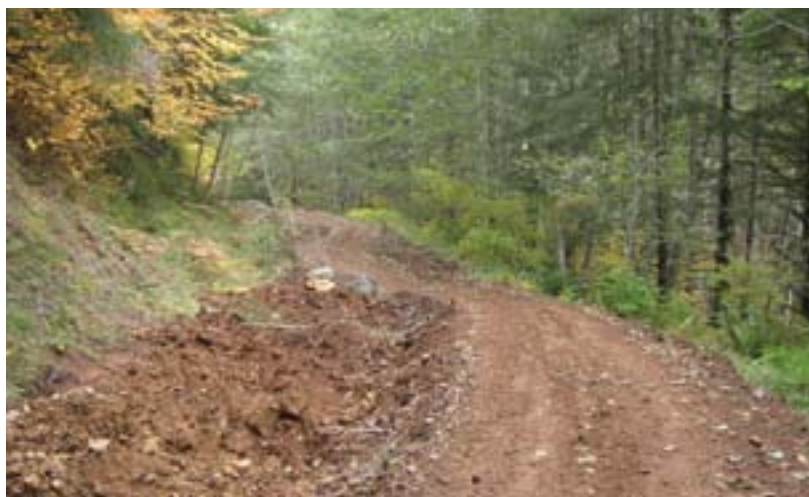
Steep, unstable ground forced the trail to stay on the existing roadbed, but the designer has created a nice sinuous flow. Ripping the unused portion of the road increases water absorption and decreases the tread watershed.
