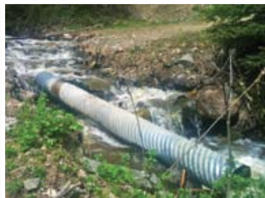
When culverts are undersized, the results can be disastrous and expensive. Spend the money up front to do it right the first time.
