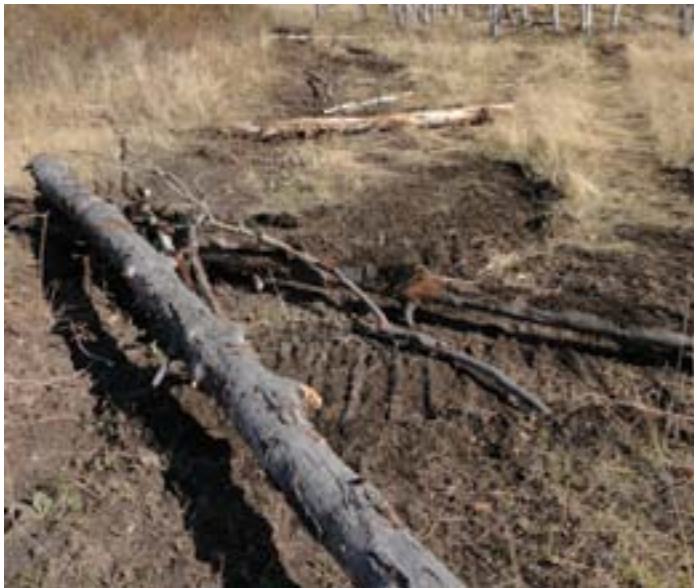
An excavator has just finished scarifying, adding drainage, and scattering debris. The project manager followed by taking down stakes and flagging and seeding all disturbed areas.
