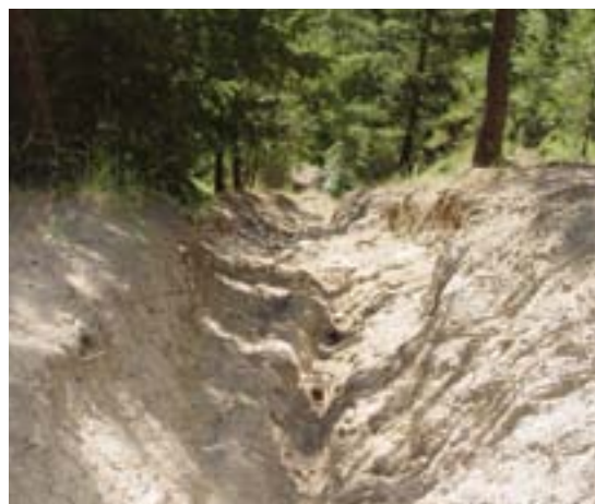
This severe erosion occurred below a road drainage point after a high-intensity thunderstorm. The sediment carried all the way to a sensitive creek below.
