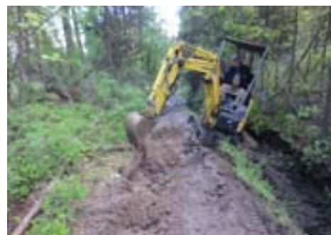
A ditch is being cut along this trail to drain the trail tread and intercept water seeping out of the inside bank. Note that the excavated material is being used to raise the elevation of the trail tread.
