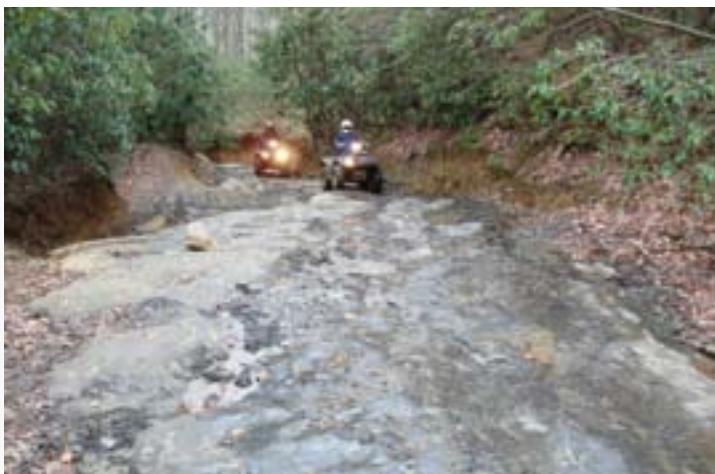
Talk about a durable tread. This trail has eroded down to bedrock, but bank erosion will still occur. Look for opportunities to drain the water off or line the bank edges with rock.
