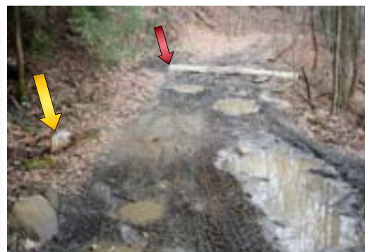
The first culvert (yellow arrow) was properly installed in the drainage. The second culvert was added later possibly to drain a spring but was not installed properly due to rocky ground. Manage your risk. The second culvert does nothing but create a safety hazard and an opportunity to ruin what was a good section of culvert. A side ditch draining into the first culvert may have been a better solution here.
