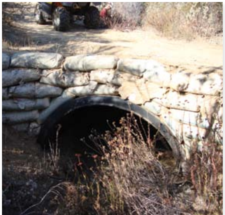
As the wrappers fall off, a premix headwall can look a little shoddy, but that is temporary. To avoid that, the wrappers can be torched off after the concrete has set.
