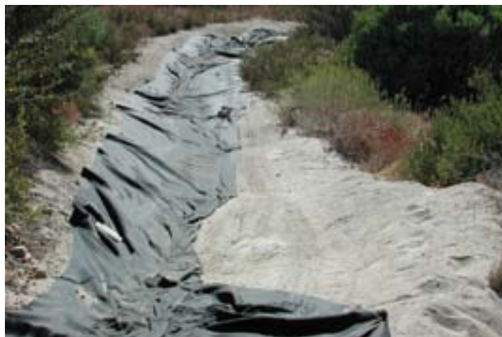
Tires and geotextile do not mix.
