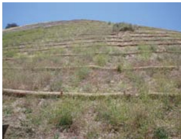
Above, rows of wattles staked closely together as part of the rehabilitation of this steep slope.
