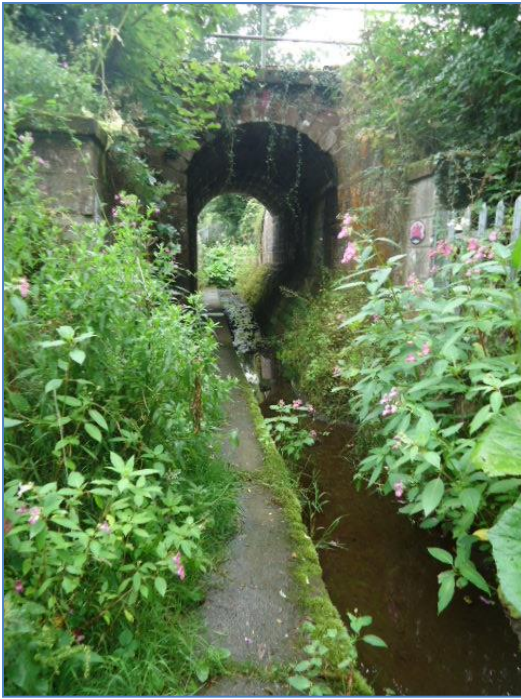
Gully under the railway
