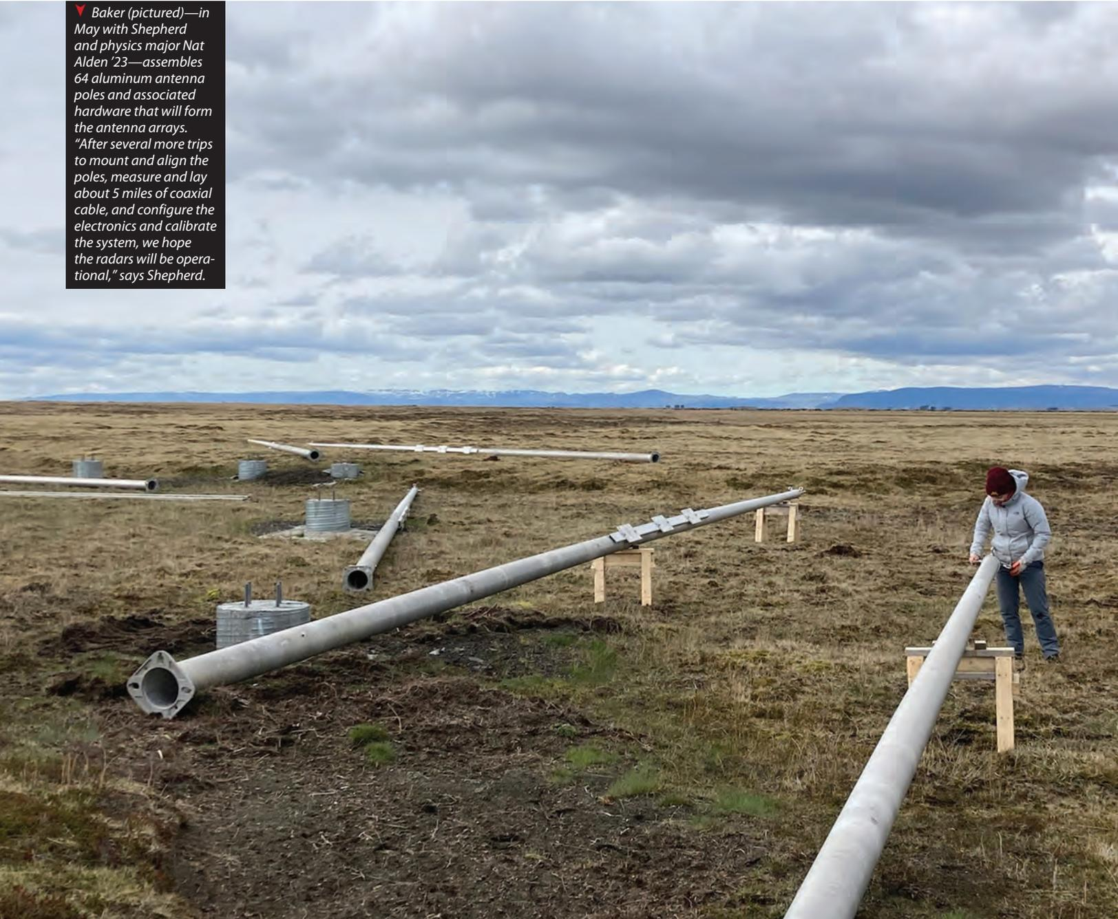
➤ With the help of a local crew during a solo trip in August, Shepherd was able to align and tension poles and begin hanging antenna wires.
