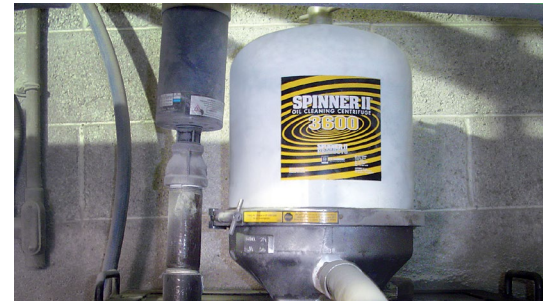
Spinner II Centrifuge mounted on crusher
