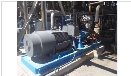
C1001020141 #2 Boiler Feed Water Pump (1-3)
