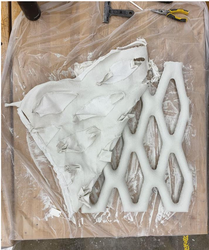
Demolding of diagrid cast with polyester jersey knit
