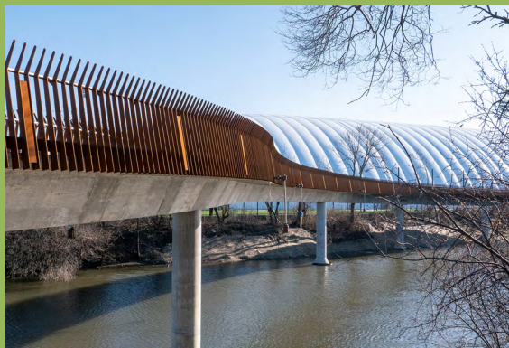
With Riverview Bridge, UrbanLab connected two public parks flanking the north branch of the Chicago River to minimize erosion and vegetation disruption on the shorefront.
